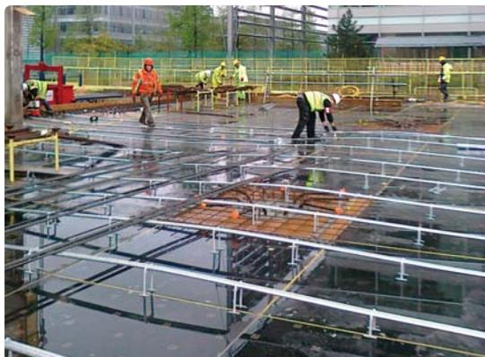
Far right: Precast edge beams with cast-in items and CCL post-tensioning duct.
