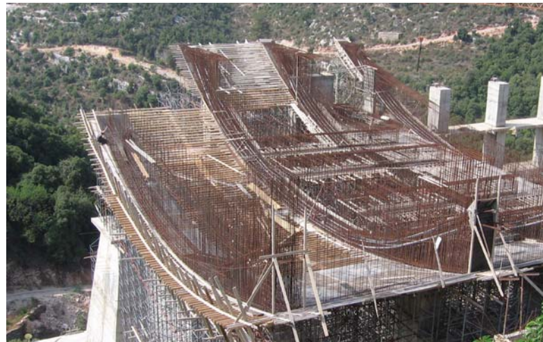
Fig. 1—One-way slab roof.
