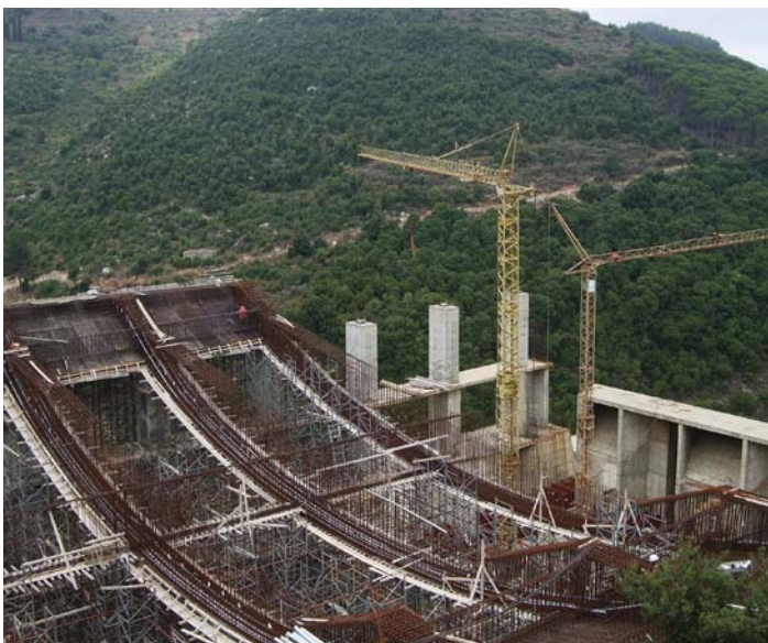
Fig. 9—Transverse beams to provide lateral resistance
