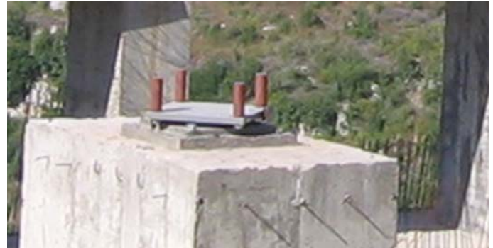
Fig. 8—CCL PG Guided Temporary Sliding Bearing.
