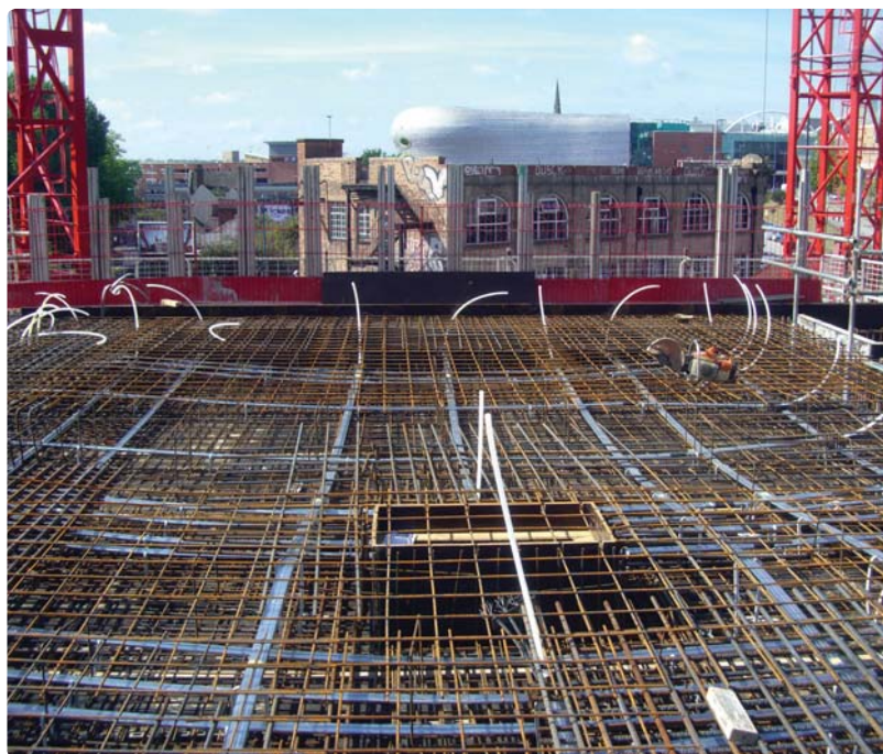
Figure 4 top left: Starter bars for precast walls and internal recess for bathroom pods.
