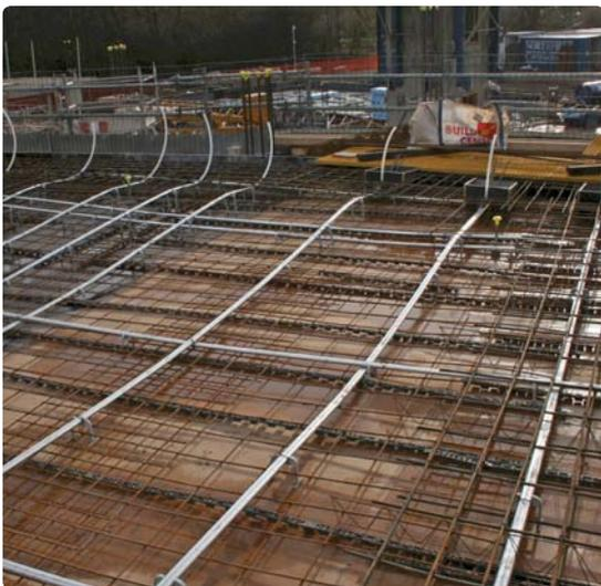
Figure 3: Bonded post-tensioning layout.
