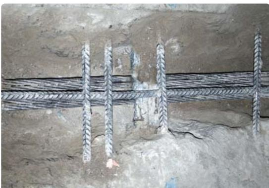
Figure 5: Exposed strand awaiting epoxy grout anchor.
