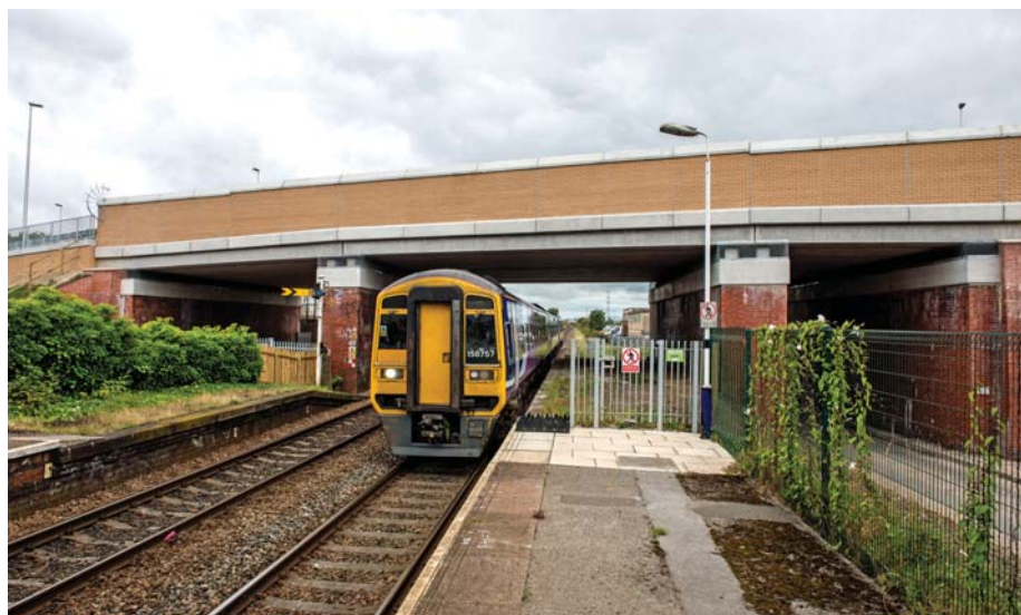
The completed three-span bridge at Plymouth Road, Blackpool.
