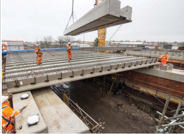
Prestressed precast beams being lowered onto CCL Elastomeric bridge bearings.
