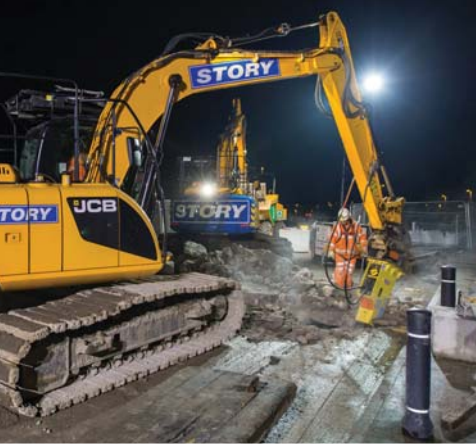
Removal of the existing three-span deck.
