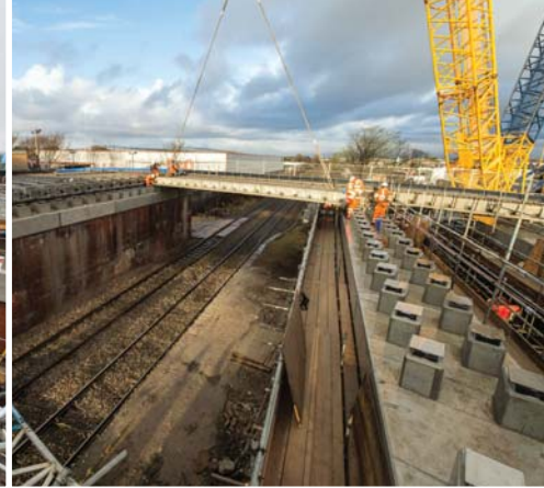
CCL elastomeric bridge bearings located on bearing shelves.
