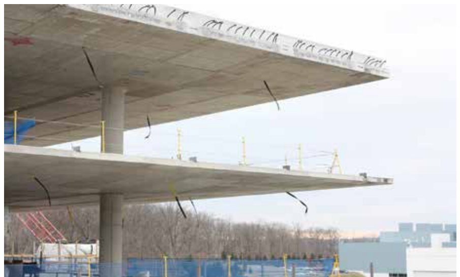
Fig. 5: View of 40 ft (12 m) cantilever at corners
