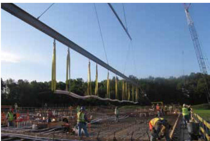
Fig. 10: Tendons were assembled and then lifted onto the slab formwork
