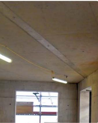
Above: Exposed soffit with rebated lighting track.
