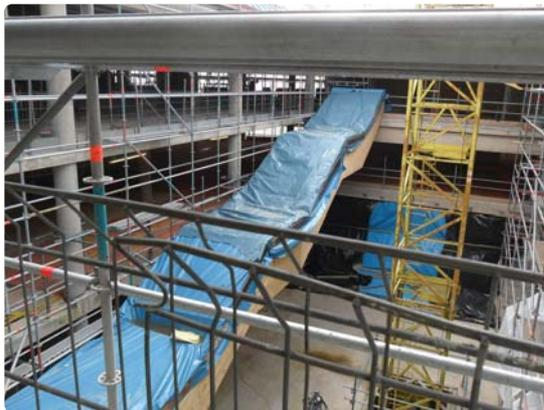
Right: Internal atrium timber feature staircase supported by cantilevering post-tensioned slab
