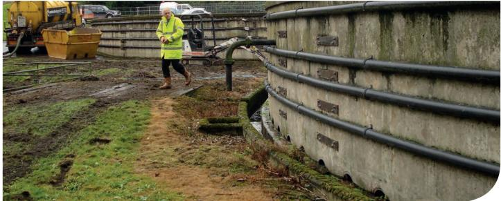
Six cylindrical concrete sewage tanks located in Dronfield, near Sheffield, required inspection in order to assess their structural condition. The tanks were constructed during the 1970s, and were beginning to exhibit signs of age.
